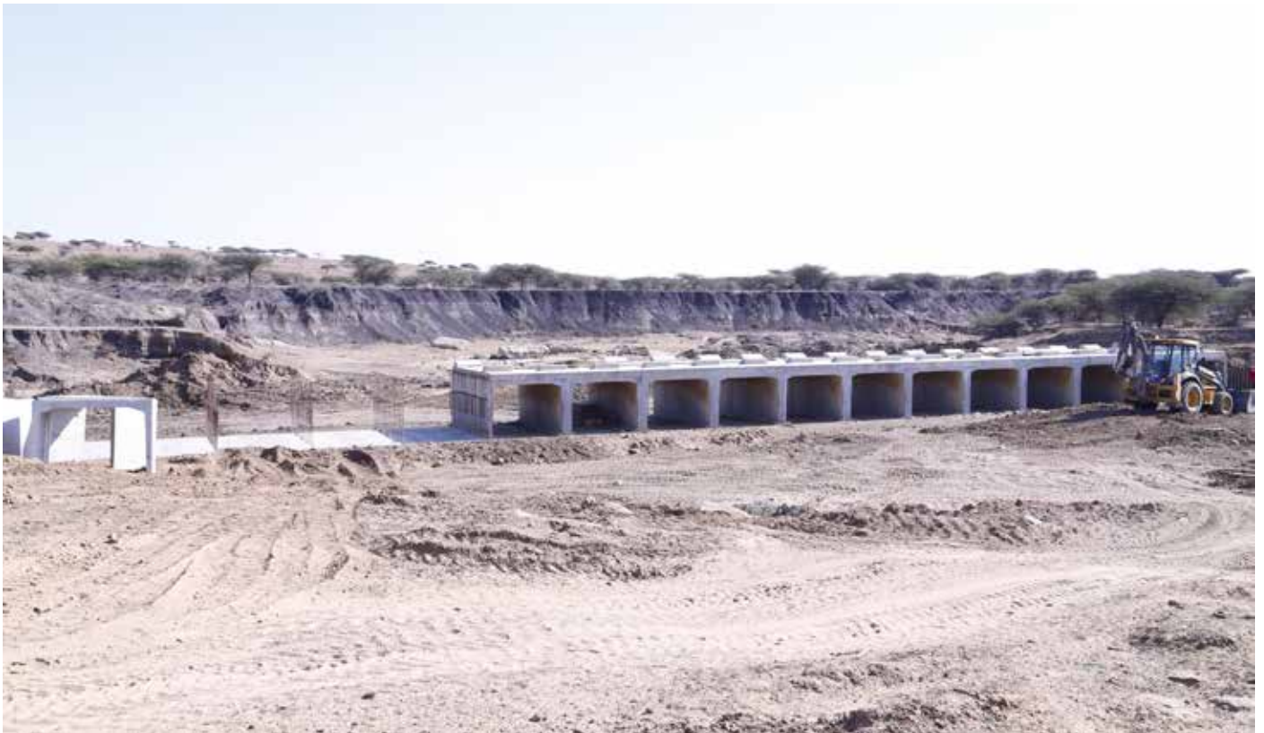
Construction of Ntinini Bridge underway in Nquthu, Umzinyathi District. PHOTOS: MBUYISELO NDLOVU
